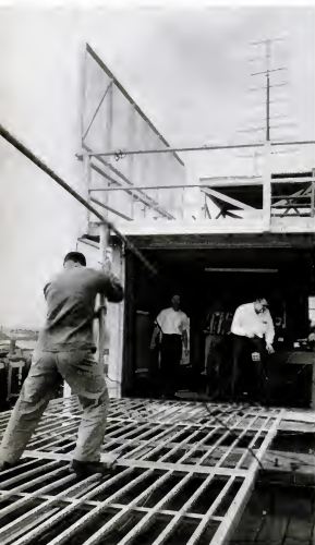
TO PICK UP SIGNALS , technicians at the Office of Naval Research lab in Washington realign a radio antenna so it will follow satellite through its orbit.
